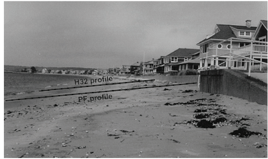
Figure 3. Photograph showing the seawall and homes that constrains the beach at Groton Long Point. The two lines show the approximate locations of the two survey transects.
